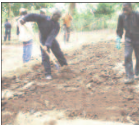
4. Contaminated soil was mixed with compost and cow manure
